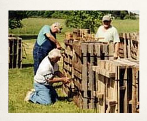
The proposed cribs are constructed of modified (slats removed) palettes. The cribs are fastened together in bundles or stacks of 5 with plastic banding. A DNR regulation requires that the cribs have a minimum of 8' of water above them so they will be placed at a depth of 12'.
